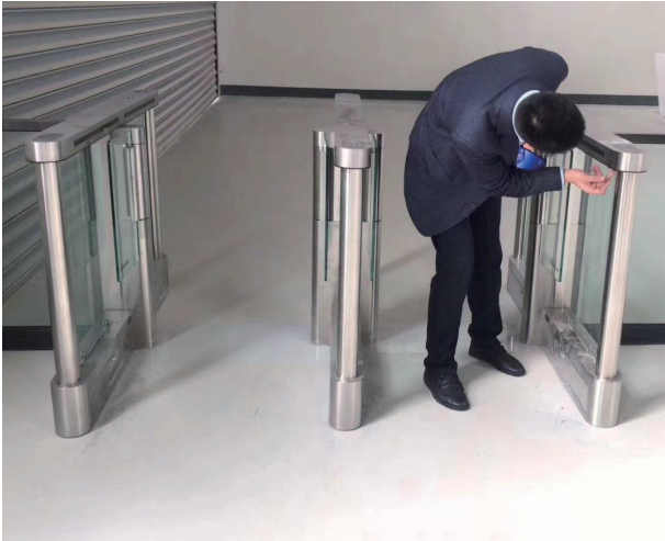
Logistics & Pedestrian Access, Building B, China Resources Phase II, Shenzhen
