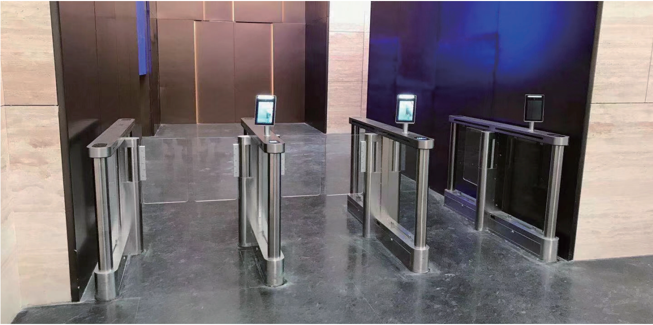
Case Study of an Undisclosed Commercial Building in Shanghai
